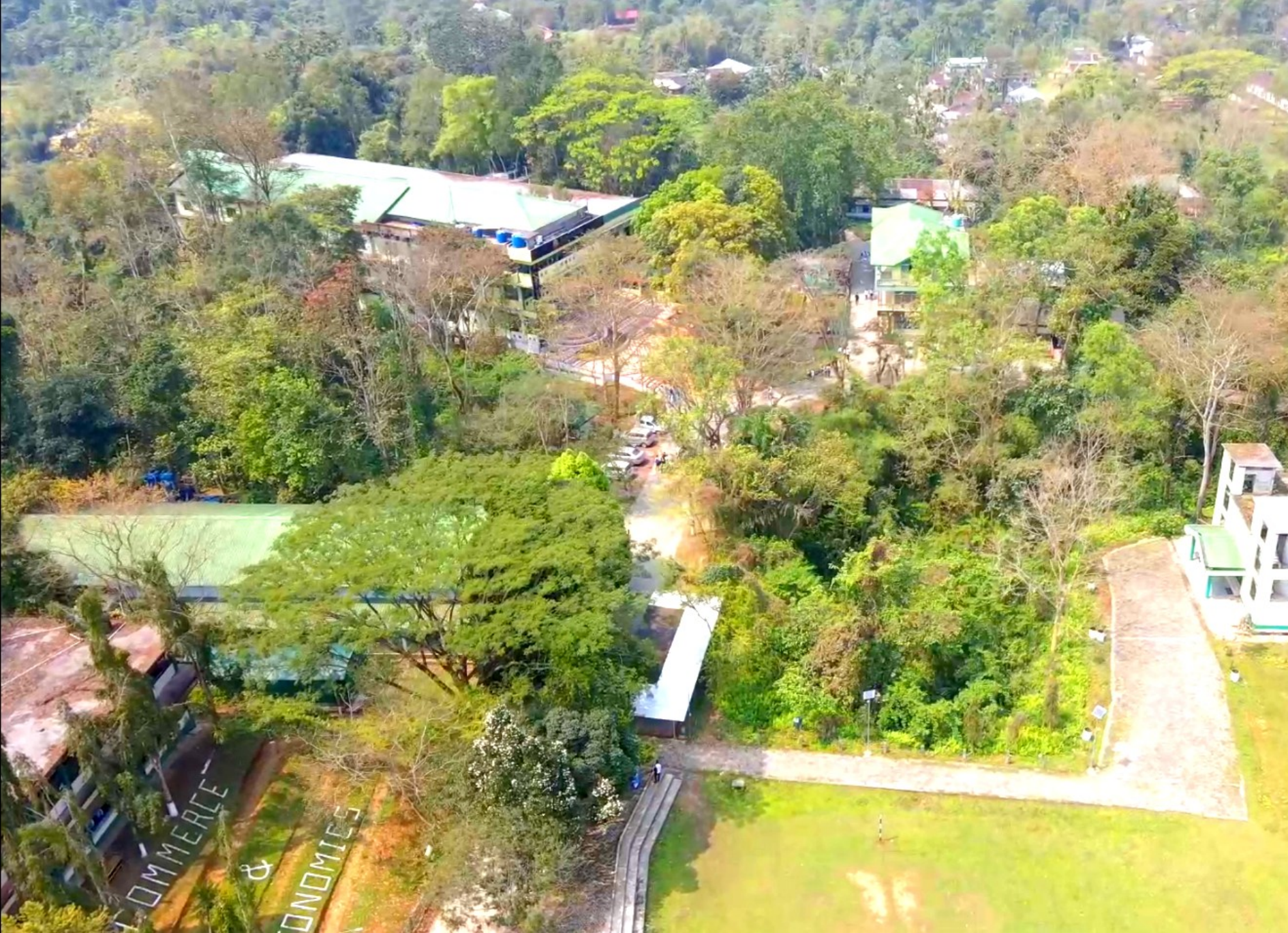
Ariel View of the Campus
