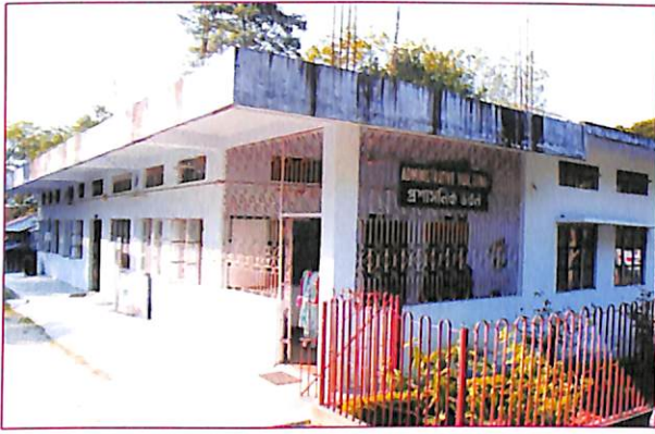
College Administrative Building
