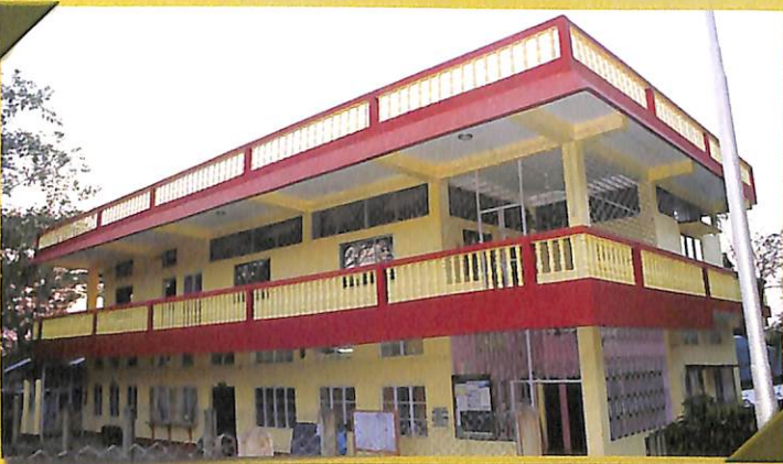
The Administrative Block of Digboi College
